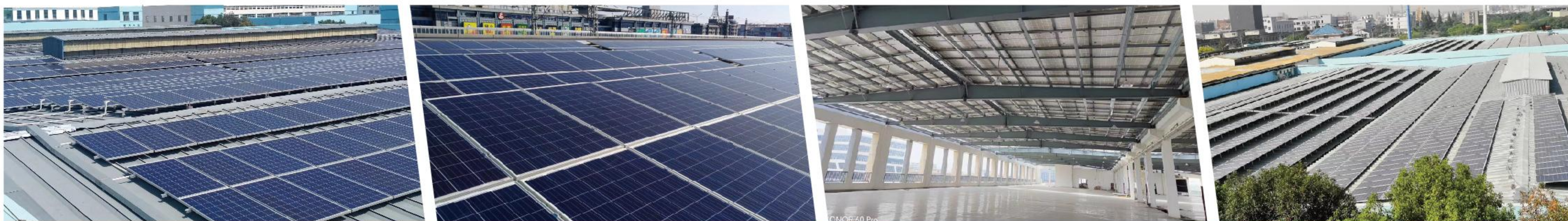
► The BAOJIANG industrial zone project in Shaoxing
