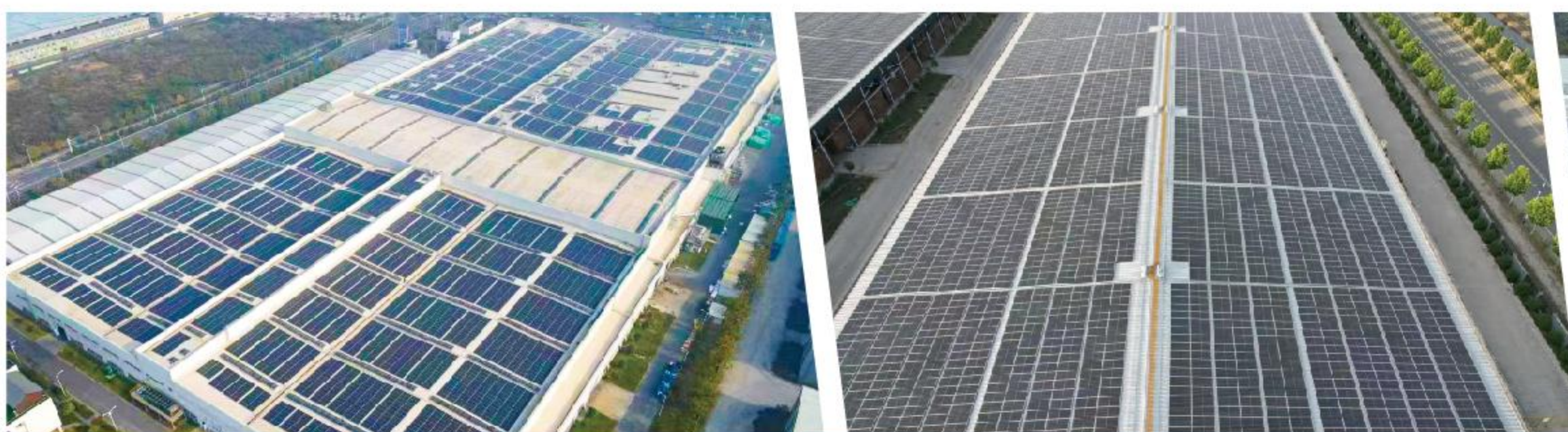
▶ Ningbo Shenzhou Textile factory roof project
