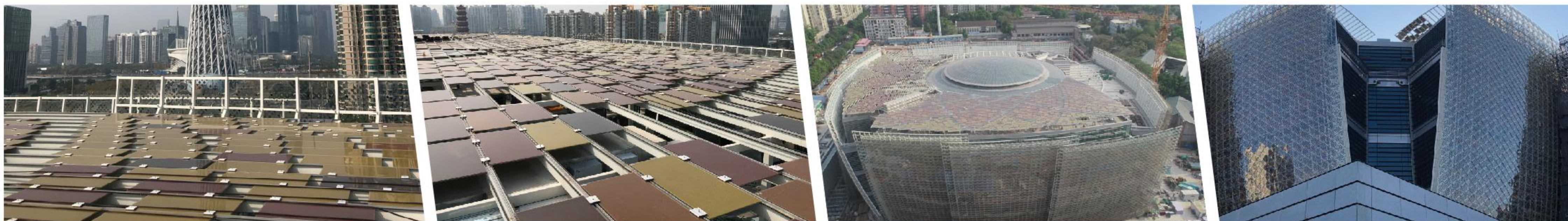
► Cadmium telluride BIPV project of Guangzhou Art Museum
